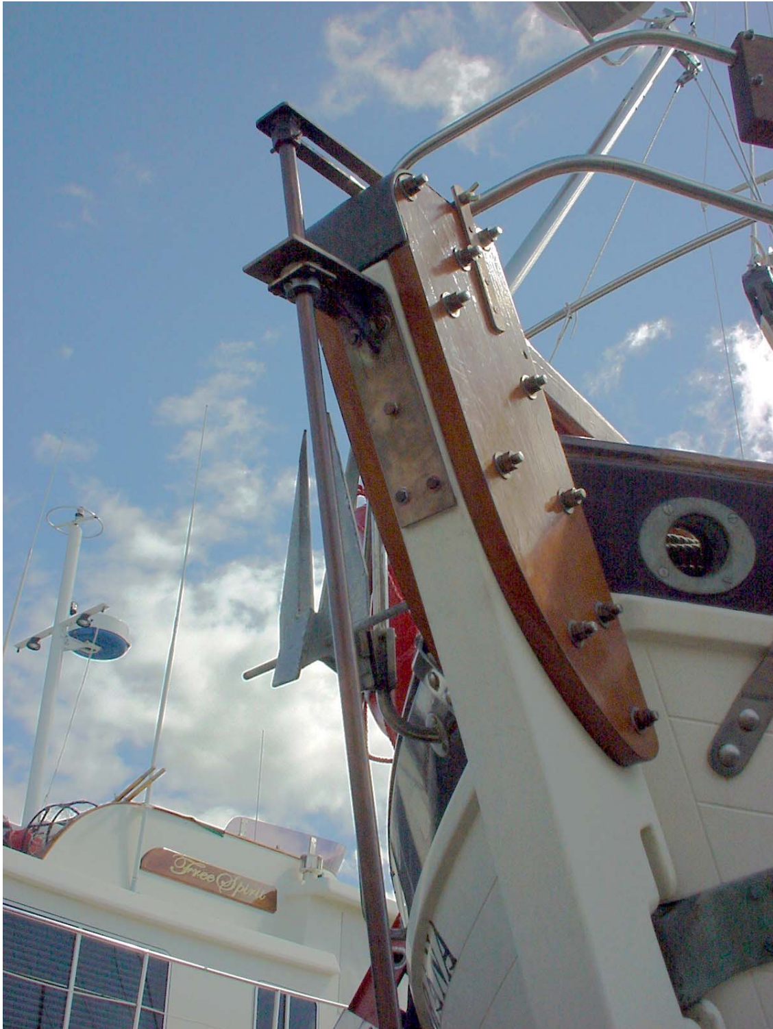
Figure 14: Above water support strut
